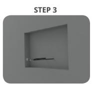
Install the cables and power supply needed for the television and ensure there is enough length to reach the connectors. Tidy any excess length away to tidy the area (power supply, HDMI, aerial cable etc).
