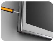
Once you are certain the television is working correctly, all the connections are installed and the screen is level, seal between the edge of the television and the wall with a waterproof silicon sealant. Ensure that any gaps are completely sealed to prevent ingress of water and dust.
